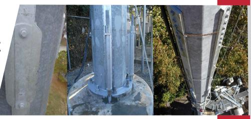
Congruex offers the telecommunications industry innovative, proprietary solutions to reinforce monopoles without the need for welding.
