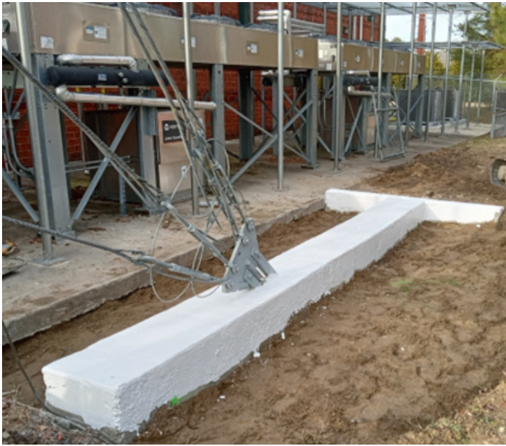
Guy-Lock™ connects new anchor shaft steel to the existing anchor head plate without disconnecting guy wires.
